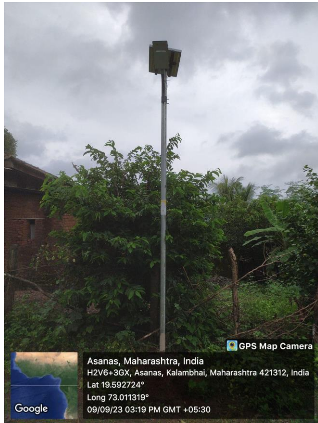
Fig 5: Solar Street light image after installation.
