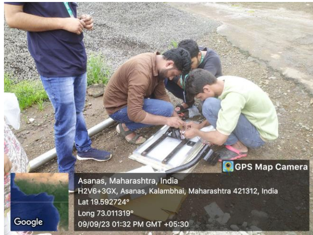
Fig 4: Students installing the Solar Street lights.
